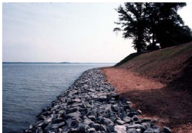
Figure I-4: Stone revetment on the Potomac River, VA
