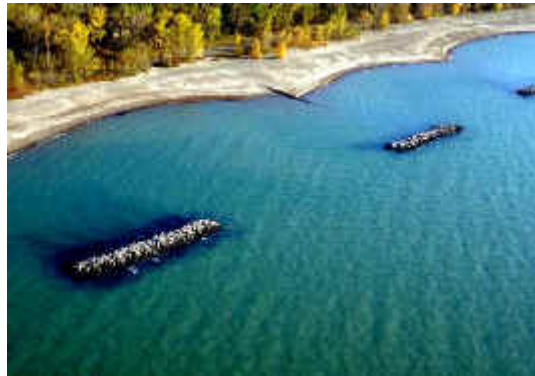
Figure I-3: A series of breakwaters
