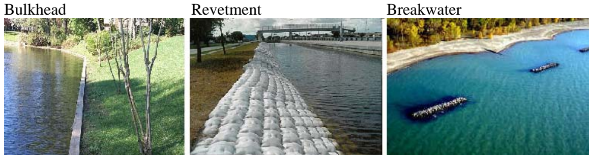
Figure I-1: Various Shoreline Stabilization Methods 1
